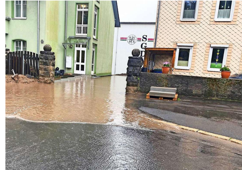
Combined Sewage Overflow in Thüringen, Germany (2021)
